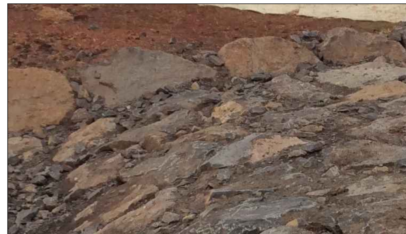
EXAMPLE OF WELL INTERLOCKED ROCKWORK WITH SEALED VOIDS
